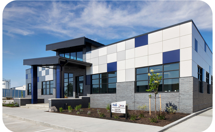
A roof over the main entrance clearly indicates where to enter the building.
