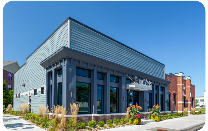
Masonry base continues around outside corner.
