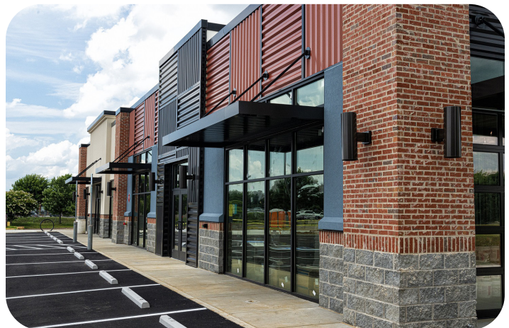
Utilizing color and direction change of a single material for a creative facade.
