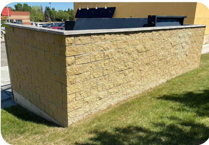
Masonry trash and recycling enclosure with coloring that complements the main building.
