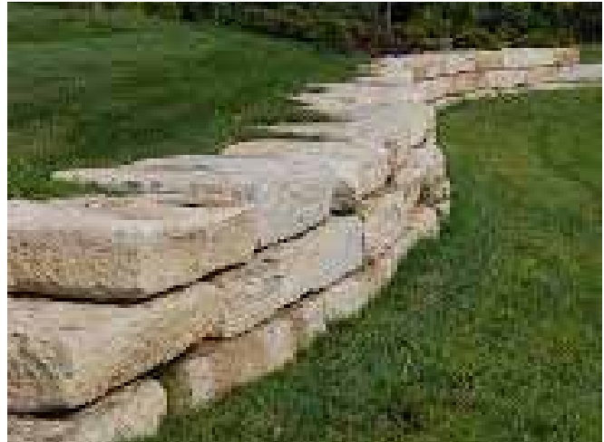
▲ Stacked limestone retaining wall
