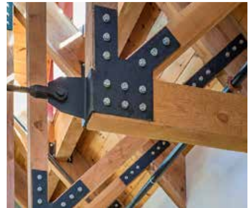
▲ Heavy timber with steel joinery. Source: vermonttimberworks.com
