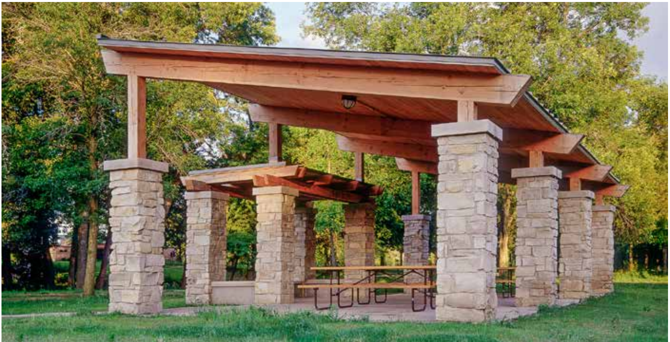
▲ Heavy timber construction can be combined with limestone foundations and post bases in pavilions and other park structures. Above a heavy timber theatre with stone post bases. Citizen’s Park in Barrington, Illinois. Source: vermonttimberworks.com
