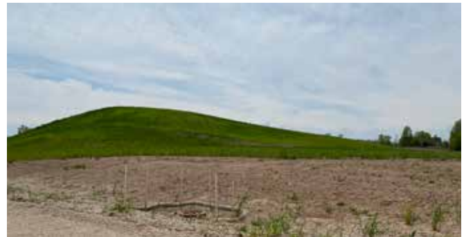
▲ Grading for a new sledding hill at Farmers Field Park
