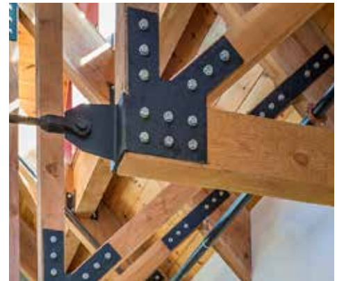
▲ Heavy timber with steel joinery. Source: vermonttimberworks.com
