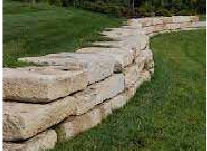
▲ Stacked limestone retaining wall
